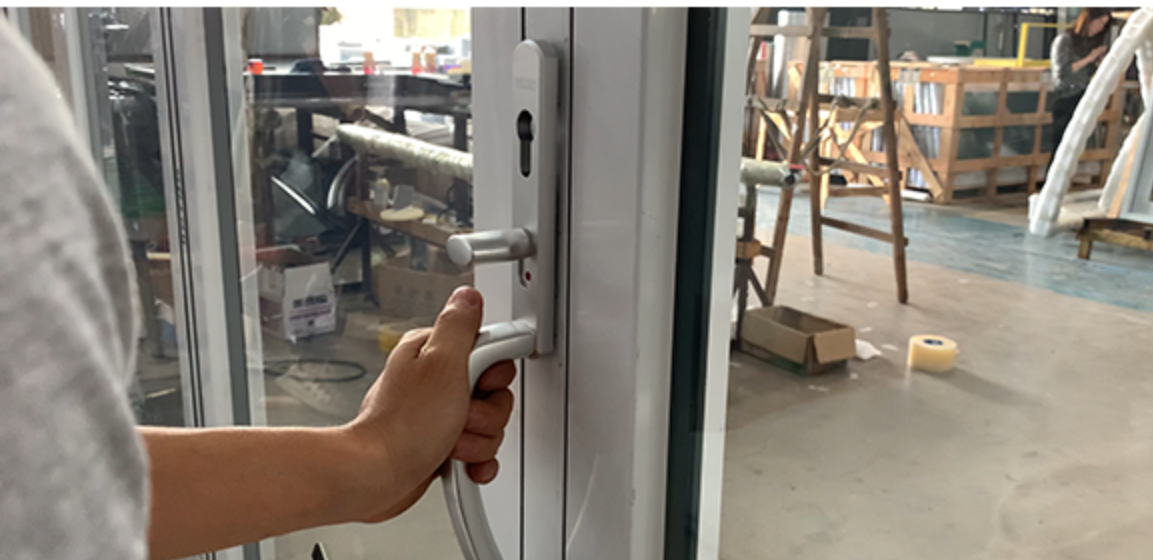
1. Put outside lock handle on holes.
