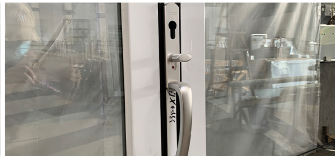
4. Align the latch with the outside lock handle hole and insert it.
