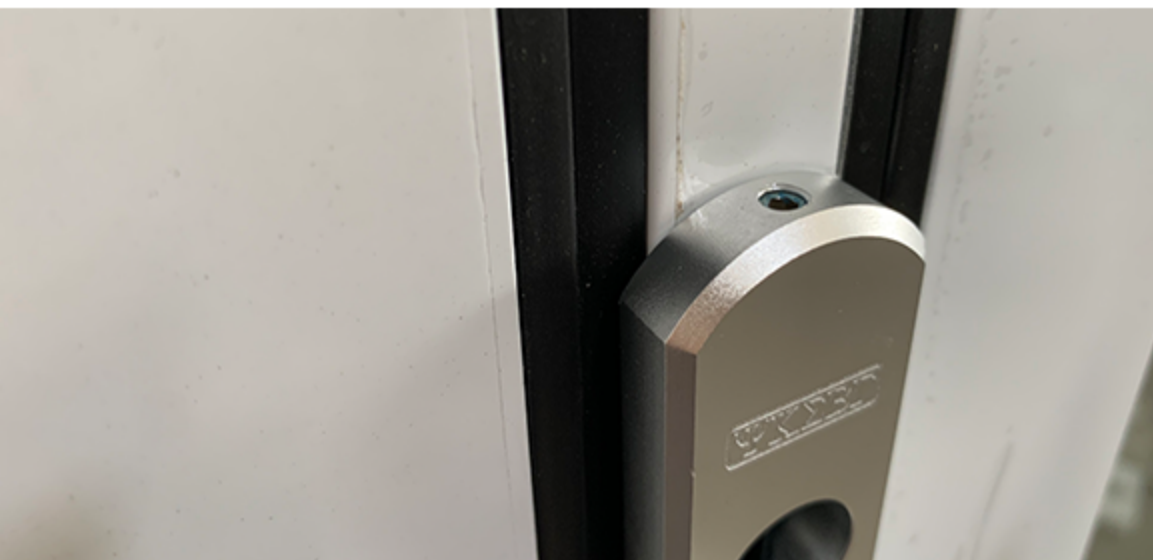
5. Tighten top hinge on lock handle.
