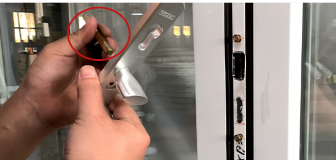
3. Insert latch into inside lock handle.
