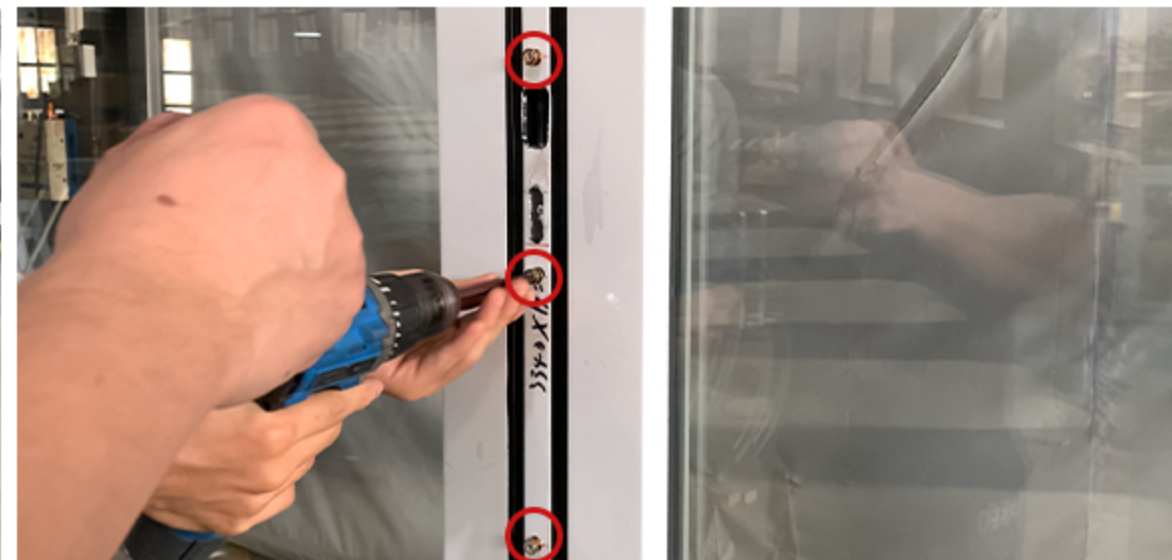
2. Screw 3 screws inside.
