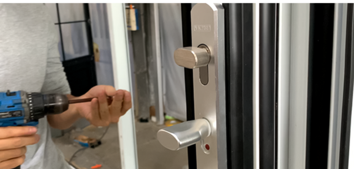
7. Insert lock cylinder into lock holes.
